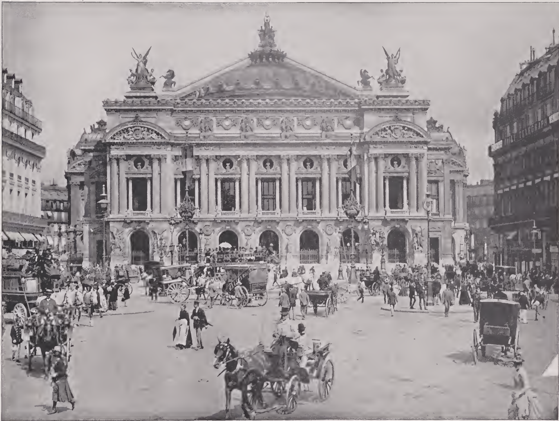
OPERA HOUSE, PARIS, FRANCE.—This is a most sumptuous edifice, completed in 1874, and covering an area of nearly three acres. Nothing can surpass the magnificence of the materials with which it is decorated, and for which almost all Europe has made contributions. Sweden and Scotland yielded a supply of green and red granite; from Italy were brought the yellow and white marbles; from Finland, red porphyry; from Spain “brocatello;” and from France, other marbles of various colors. The cost of the site was over $2,000,000, and that of the building nearly $8,000,000.
